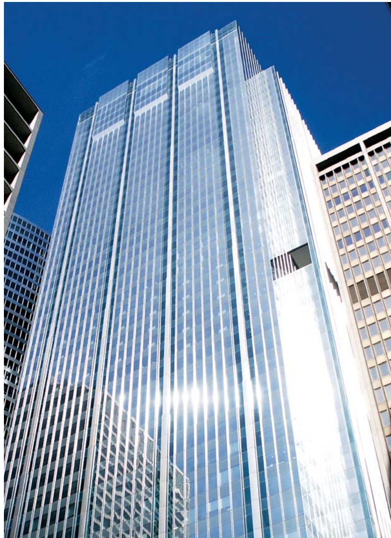
Thermafiber® Safing and FireSpan® mineral wool products provide the critical components of the perimeter fire containment system in the 111 South Wacker Building in Chicago, IL. Thermafiber® mineral wool insulation also contributed to the building's LEED® Gold Rating.
