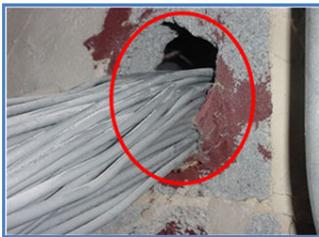
Of all leaks, cable trays and conduit paths are notoriously difficult to seal, especially once cables have been installed, and can often mean the difference between an enclosure that passes and one that fails the enclosure integrity test. This is especially true for small rooms and data closets that rarely pass the enclosure integrity test.
